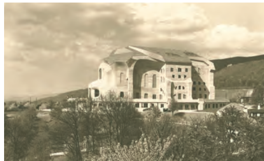
The second "Goetheanum": flowing reinforced concrete.
